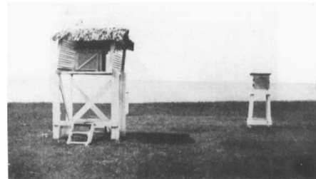
Figure 10. Tropical and Stevenson screens at Apia, Samoa (from Sapsford, 1940). © SIR Publishing, Wellington, New Zealand.
