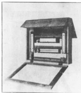
Figure 4. Thatched shelter and associated thermometer cage for use in the tropics (from Field, 1920) © HMSO
